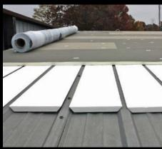
RhinoBond is also an ideal option for metal roof retrofit applications. Because the system does not require in-seam fastening, the membrane seams do not have to be positioned over the purlins. This eliminates the need for specialty purlin-width sheets, simplifies the installation and reduces waste.
